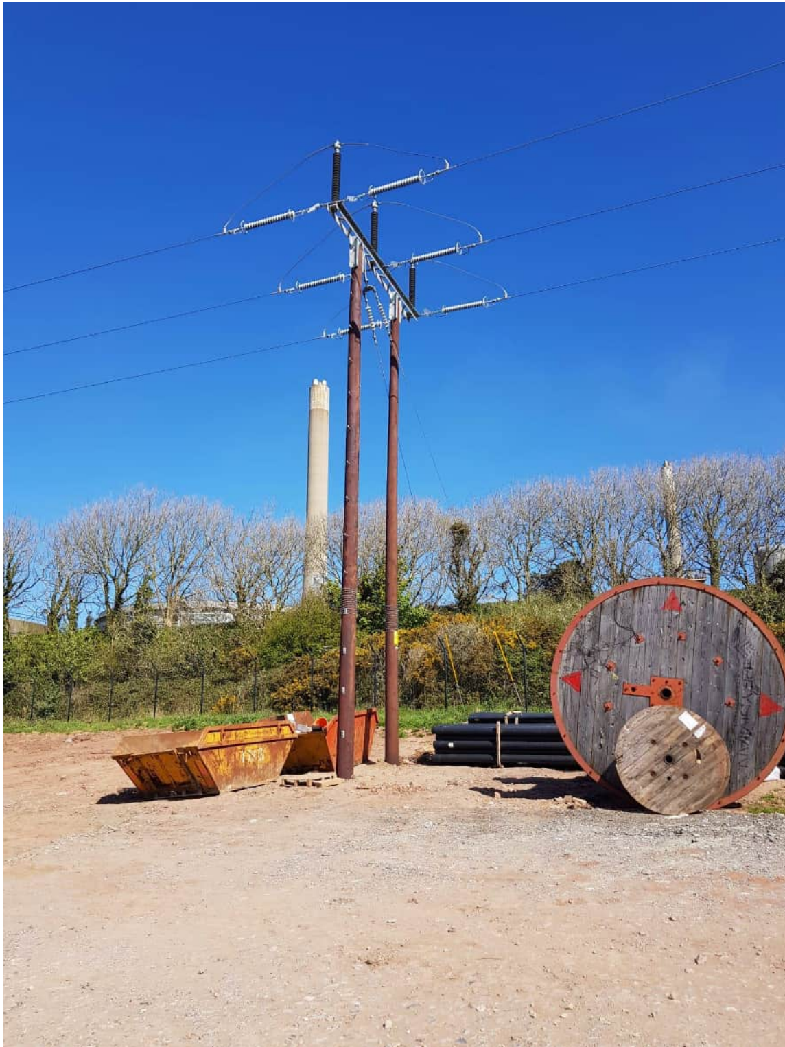
Figure 1-3 - Intermediate Overhead Line (H-Pole)
