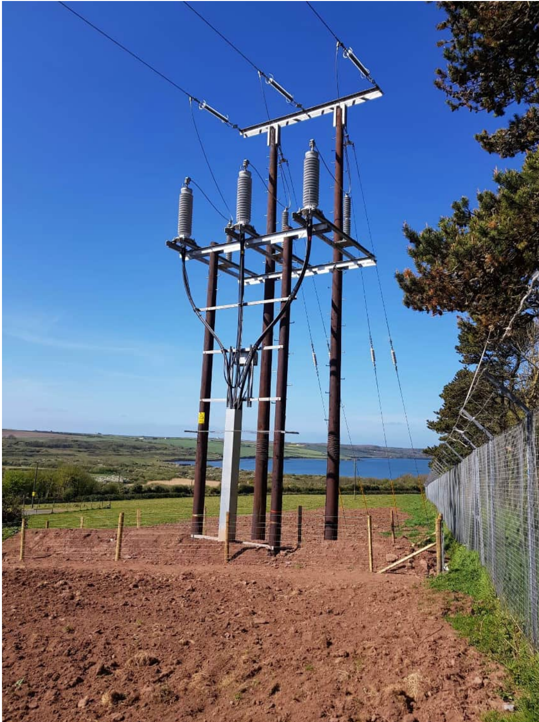
Figure 1-4 - Overhead Line to Underground Cable Terminal Connection Point (H-Pole)
